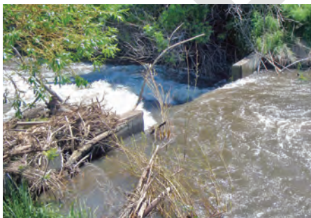
Stream Barriers to Fish Passage. The 73 identified barriers restrict passage connectivity either at a specific life history stage or seasonal flow condition. Although the potential barriers don't appear to be restricting a significant extent of the historic range, they do have an effect on the population by restricting the migration patterns of juvenile life history stages.
